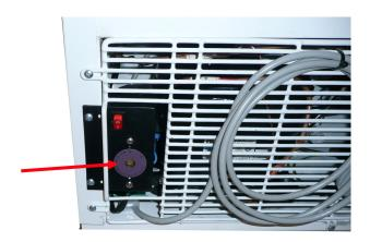
The temperature can be adjusted by using the thermostat button at the back of the cabinet. Set to position 5 on the thermostat scale. Place a thermometer approx. 10 cm inside the cabinet on the top shelf and check the temperature once it has achieved steady conditions. Turn the thermostat button clockwise if the temperature is too high or anti-clockwise of the temperature is too low.
